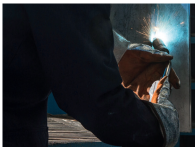
All position welding
