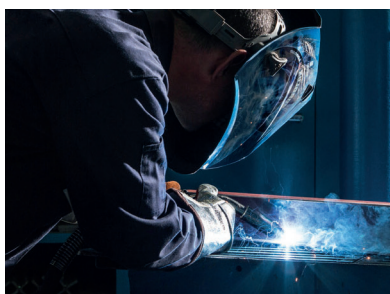
Manual MAG welding
